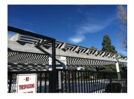
**Description:** Wood framed shade pergolas with cedar boards, posts, joists, and beams.
