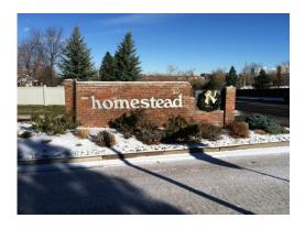
**Description:** 1 foot wide brick walls with varying height and length. Monuments have metal lettering attach to the brick walls (both sides) that say "homestead" and have metal section with a tree cut out from it. 4 brick monuments have no lettering but have a black metal section with a tree cut out from it. Each monument area is vegetated with grass and/or plants. Entrance monument on South Jersey Street has a partial rock wall veneer on the base of the monument island.
