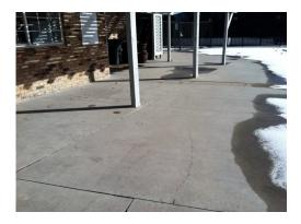
**Description:** The pool deck is made of a cast-in-place, on-grade, and reinforced concrete slabs.
