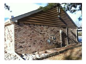
**Description:** Painted hardboard lap siding, typically installed over building paper or other water resistive membrane and attached to the wall framing. Hardboard trim material installed around windows, doors, and creating the soffit and fascia details for various roof eave pool house overhangs.
